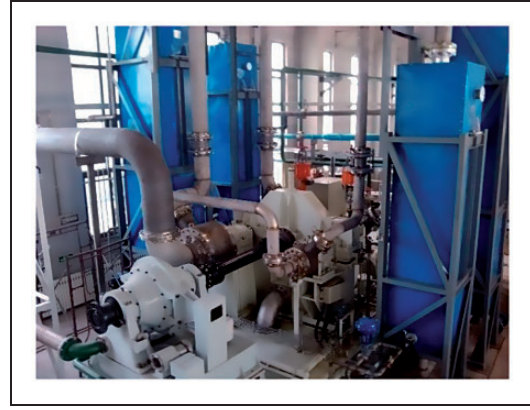
Figure 1. Four-stage reheating radial inflow turbine.
