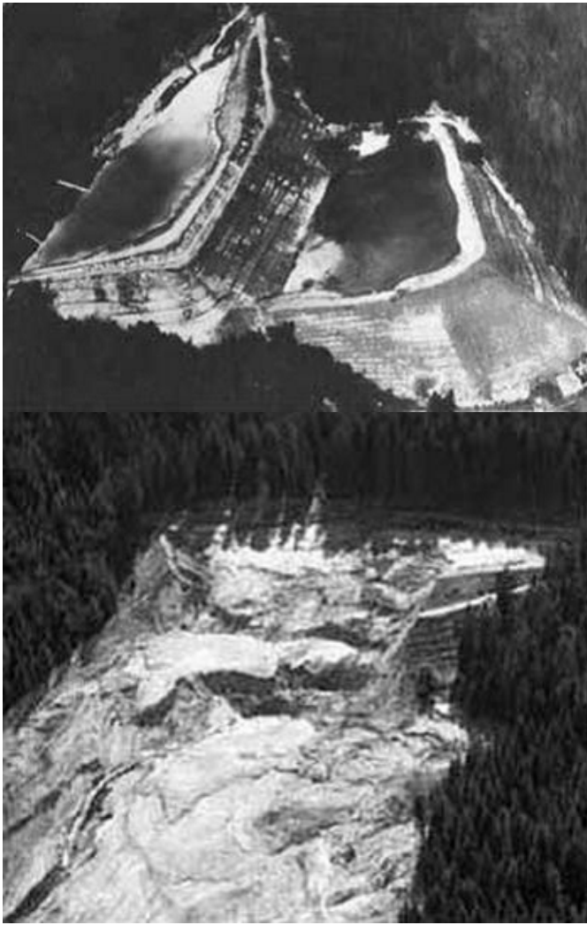
Figure 2 – The Stava tailing basins before (upper) and after (lower) collapse ( http://www.stava1985.it )
