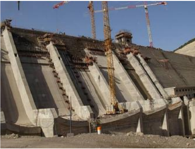
Figure 4. Koudiat Acerdoune under construction
