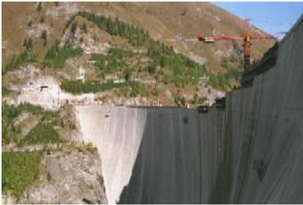
Figure 8: Luzzone Dam raising works
