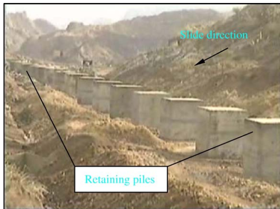
Fig. 10. Stabilizing piles for landslide control.
